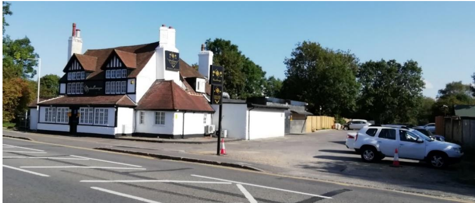
Photograph 2A: the rear elevation of the lounge area of 74 Oxford Road
