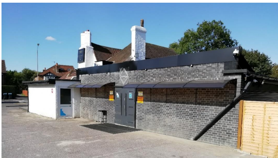
Photograph 3: the side entrance the structure
